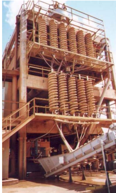
Figure 2. Itamarati de Minas' preparation plant
